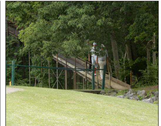
The cool trestle bridge on hole #2 crossing the 'gorge.'
